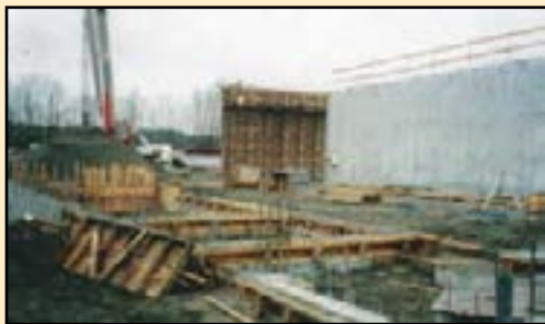
Construction of Burnaby Mountain Secondary School
