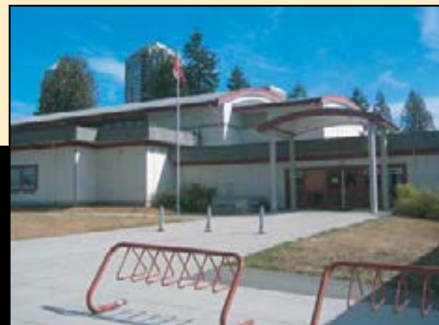
Taylor Park Elementary School
